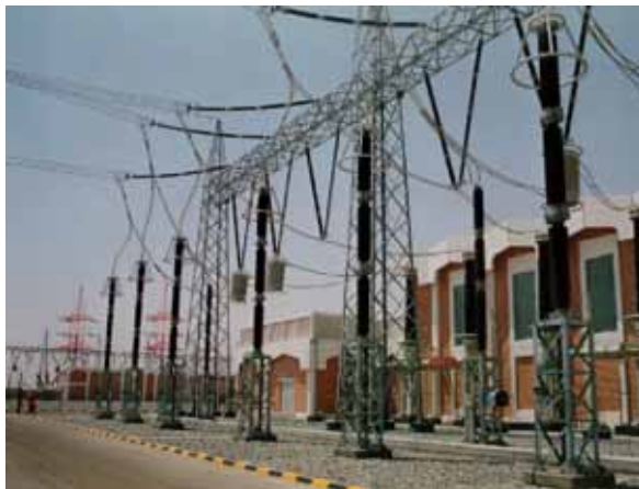
In a 420kV system, Pollution Level = 60mm/kV (1994)
